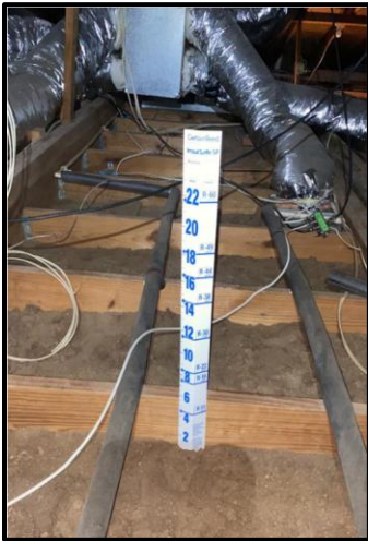
Pre-install Representative Area
