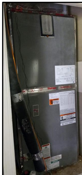
Indoor unit (electric resistance)
