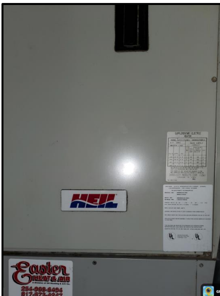
Indoor unit (electric resistance)
