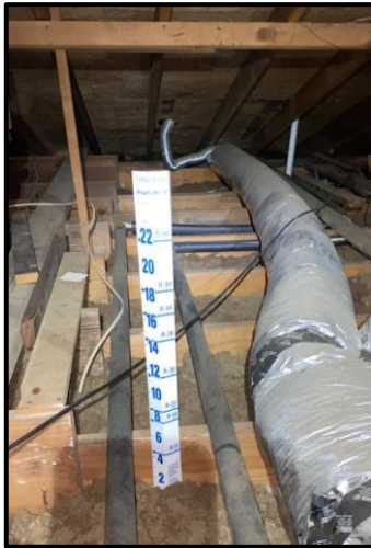
Pre-install Representative Area
