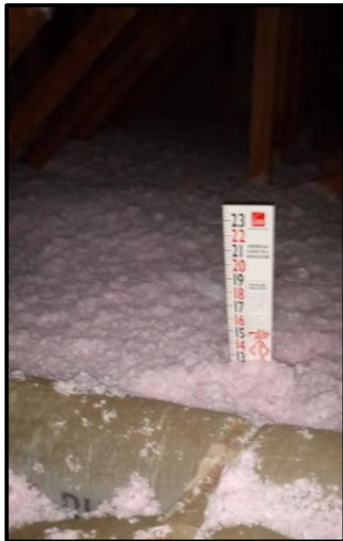
Post-Install Representative Area
