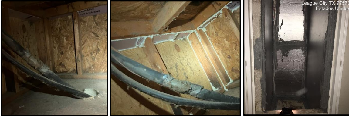
Supply air plenum before and after
