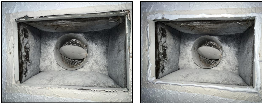
Supply register in home before and after
