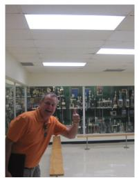
The Santo Independent School District recently replaced all of its old fluorescent lighting (34-watt T12, magnetic-ballast) with new, energy efficient T8s (28-watt lamps, with instant-start, electronic-ballasts).
